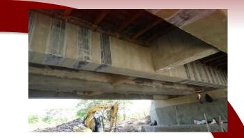
Composite materials comprised of continuous fibres in a polymer (FRP) or, more recently, cementitious matrix (FRCM), are a satisfactory technique for increasing the durability and performing rehabilitation solutions in existing structures. Debonding from substrate and shear strengthening of reinforced concrete (RC) with FRP and FRCM are the main topics investigated in this research project.
